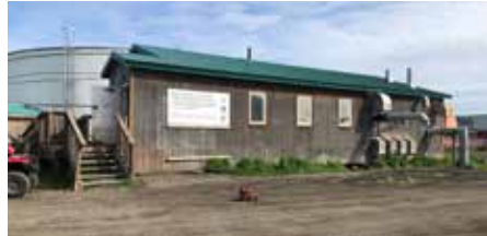
The Stebbins Washeteria's rehabilitation is among a long list of regional projects vying for funding.
