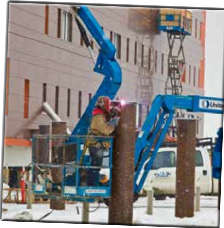
A piling is welded outside where the ER entrance was built
