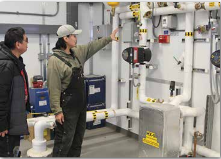
WATER PLANT TOUR Richard Kuzuguk, NSHC RMW program manager, and George Otten, Stebbins water operator, tour Stebbins' relatively new water plant, which hosts a recycled heat system that supplies heat to several public buildings in the community.
